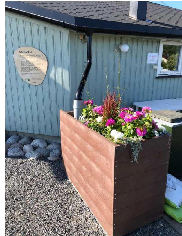
Marmax Raised bed raingarden [SUDSBOX ] in Oslo, Norway 2019. In the UK there is the same need, but is there a market? Additional options needed too.
