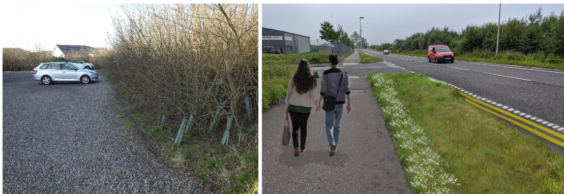
Kerbs or hedgerows as physical barriers to runoff? Willow swale at Dance Connect . Retrofit options for keeping vehicles out of swales: add rumble strip and double yellow lines? (snow-drops for early spring enhancement shown too?).
